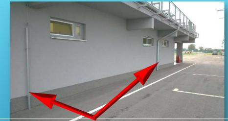
Use the lightning conductor for grounding Wire between exhaust and lightning conductor is enough.
